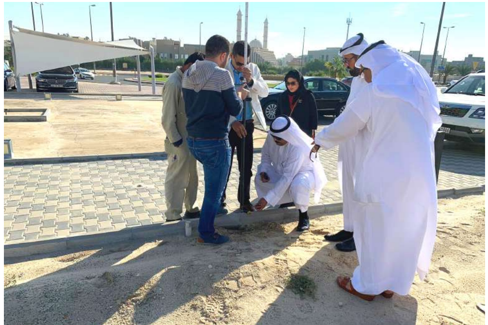
Figure 1: Surveyors and municipal officials mark an encroachment. By combining precise measurements with cadastral data they can quickly identify any problems.
