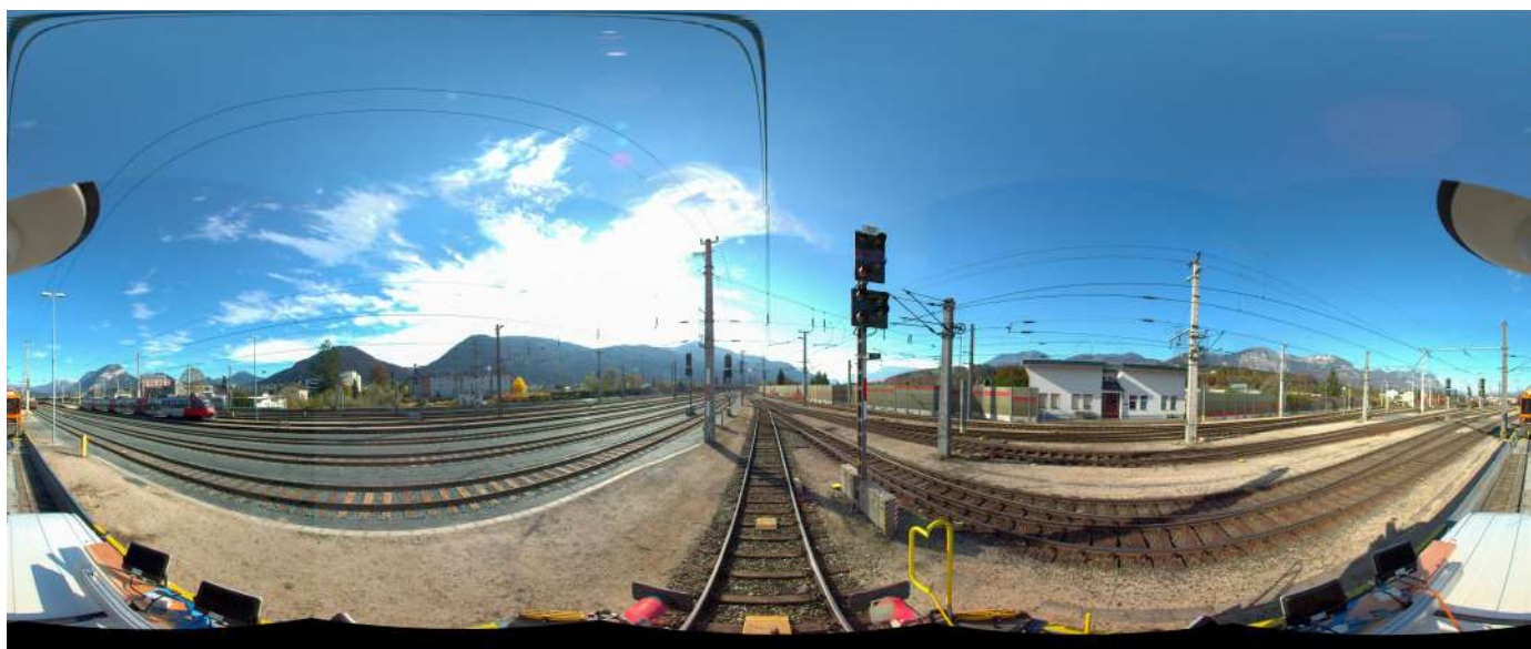
Figure 4 (top) & 5 (bottom): The MX7 captured a 30MP panoramic image every 4 m along each of the tracks and acquired important features such as switching boxes that were not visible in the aerial photogrammetry.
