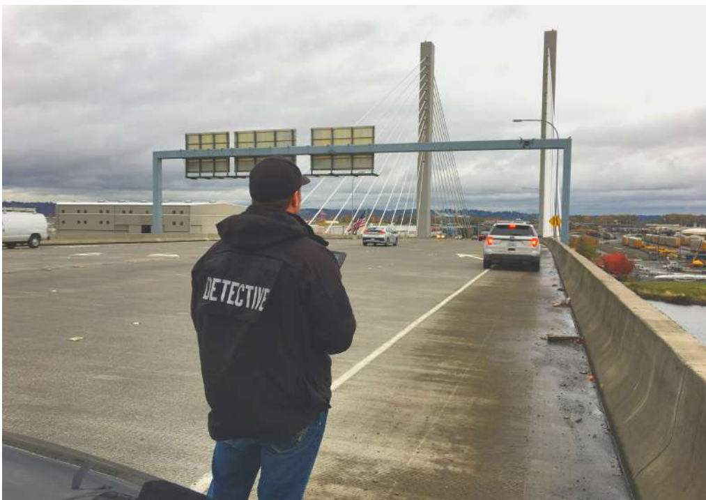
Figure 7: Det. Gunderson operates the WSP’s Matrice 200 UAV.
