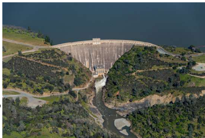
Figure 1. Pardee reservoir across the Mokelumne River, California
