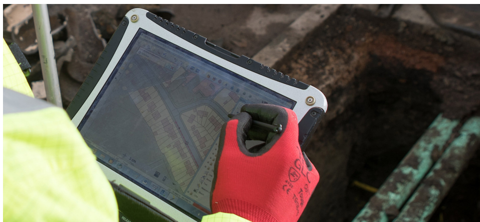
Figure 1. mobile solution that uses high-precision GNSS equipment to measure and map the exact coordinates of each new pipe as it is laid
