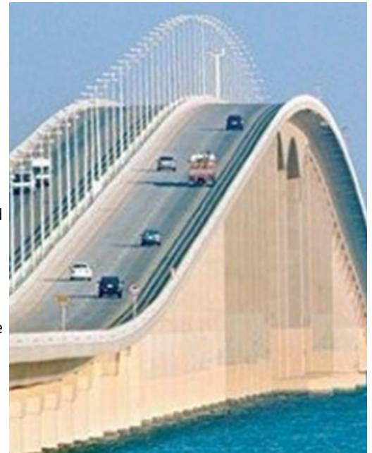
Figure 4. A portion of the King Fahd Causeway, connecting Saudi Arabia and Bahrain. The five dual, individual pillar supported bridges have Trimble Monitoring Solutions systems installed for real-time monitoring.
