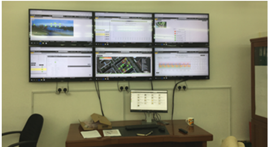
Figure 7. A user control center, which enables users to easily view and visualize real-time data. This is the King Fahd Causeway control center.
